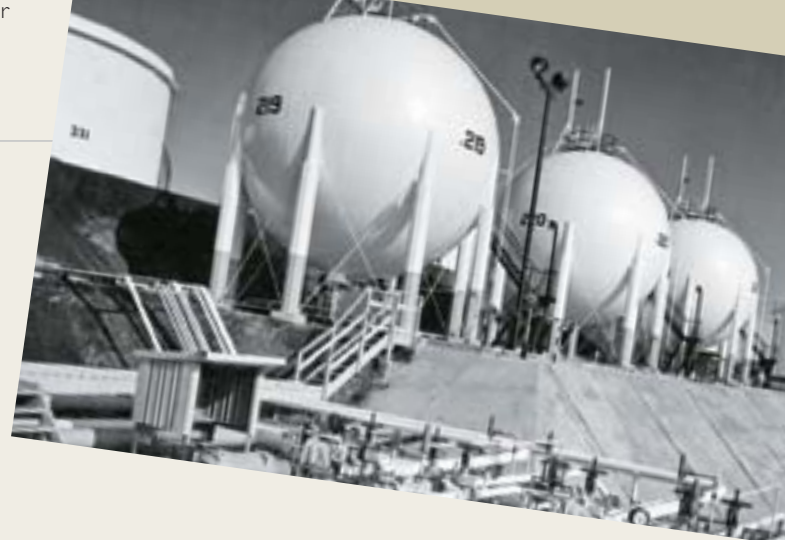
BELOW These three 9.8 metre diameter spheres are designed to hold up to 453,000 litres of butane each. Butane is used as a component of petrol and autogas, and as an industrial fuel.
