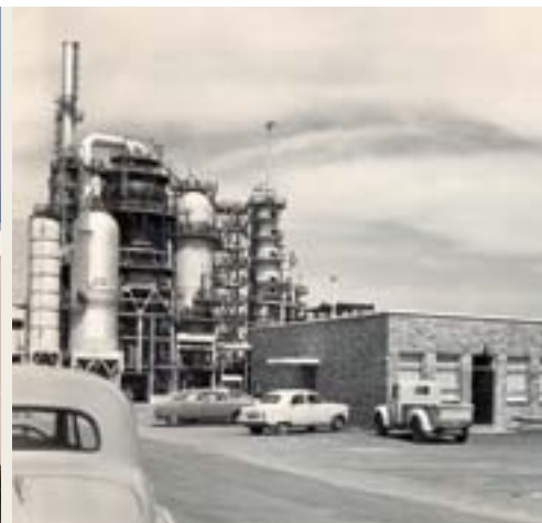
ABOVE LEFT There are more than 100 petroleum product and crude oil tanks at the Kurnell refinery which hold an inventory of up to 600 million litres. Today the refinery processes around 26 million litres of crude each day, a dramatic increase on the 4 million litres a day throughput in 1956. RIGHT One of the original plants that went online 50 years ago was the no. 1 fluid catalytic cracking unit at Kurnell. It continues to produce petrol today.
